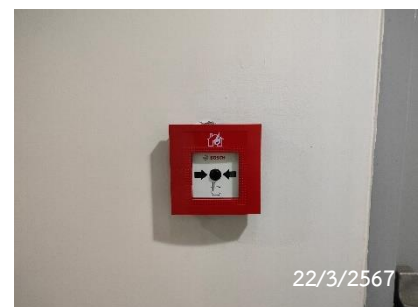
Fire Alarm Manual Station
