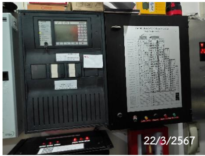
Fire Alarm Control Panel
